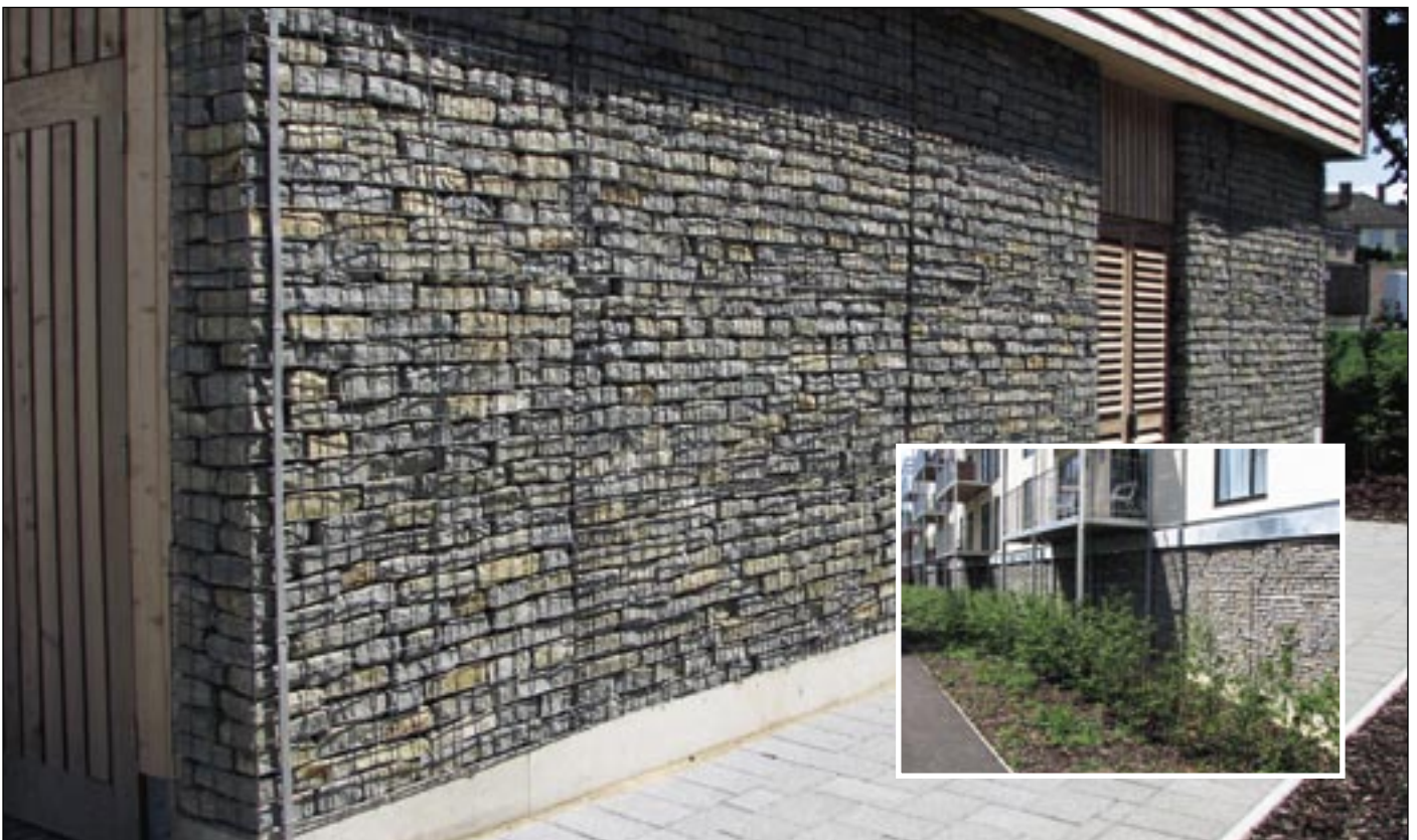
▲ Gabion 27 System cladding to a new build at Street, Somerset.
