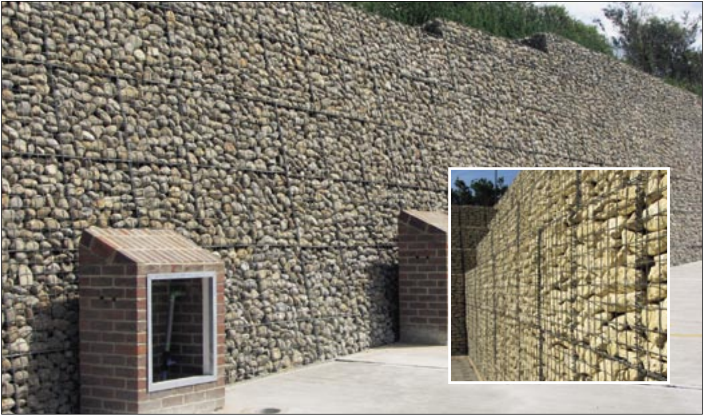
▲ Gabion 27 System wall, designed and constructed at Bridies Tan, East Sussex.
