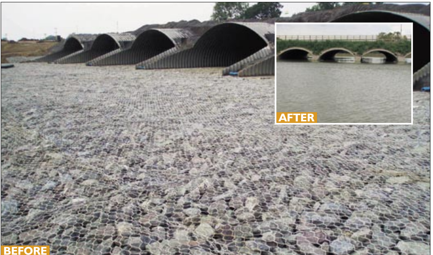
▲ Hexagonal woven wire mattresses acting as an erosion protection apron to a new lagoon at Swann Valley, Northampton.
